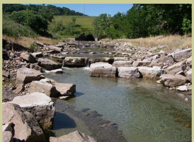
West Creek Downstream of I-480
