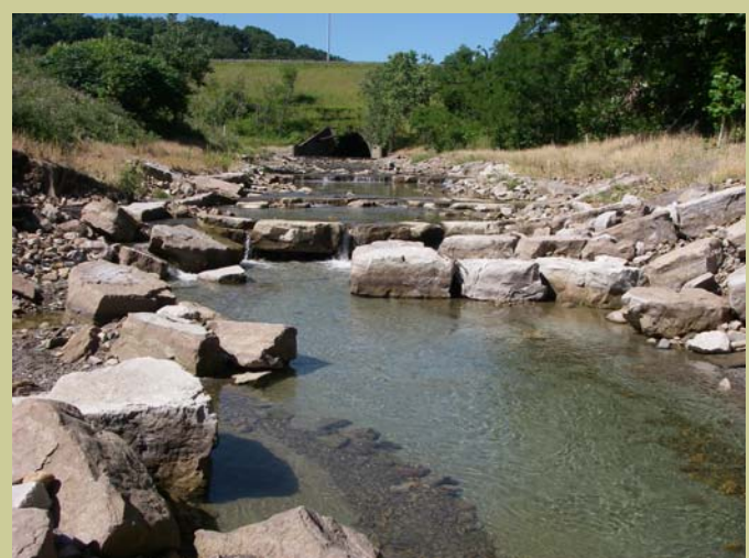
West Creek Downstream of I-480
