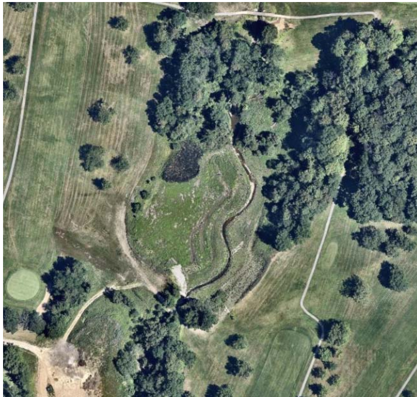
Figure 3. Constructed wetland depression in place of drained pond (2017)
