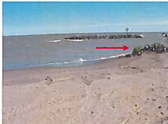
SAMPLE SITE Pile of stones
