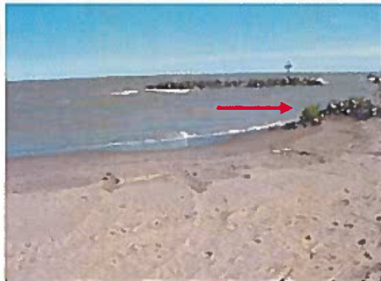
SAMPLE SITE Pile of stones
