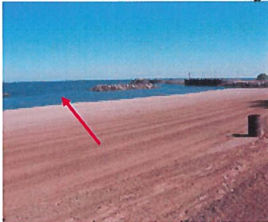
EAST SAMPLE SITE Mid-distance between 3 rd and 4 th break walls
