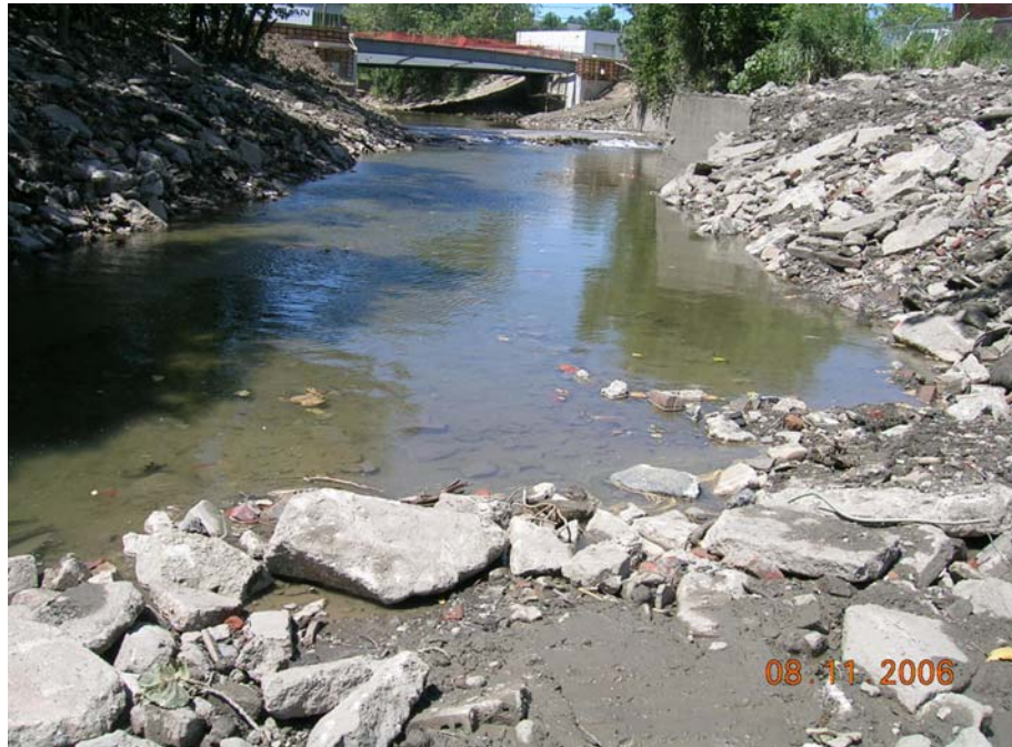
Figure 3. Jennings Road bridge during construction.
