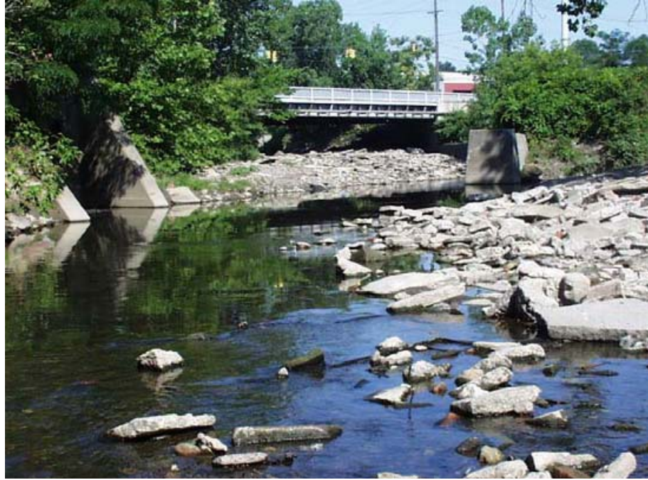
Figure 2. Jennings Road bridge prior to construction.
