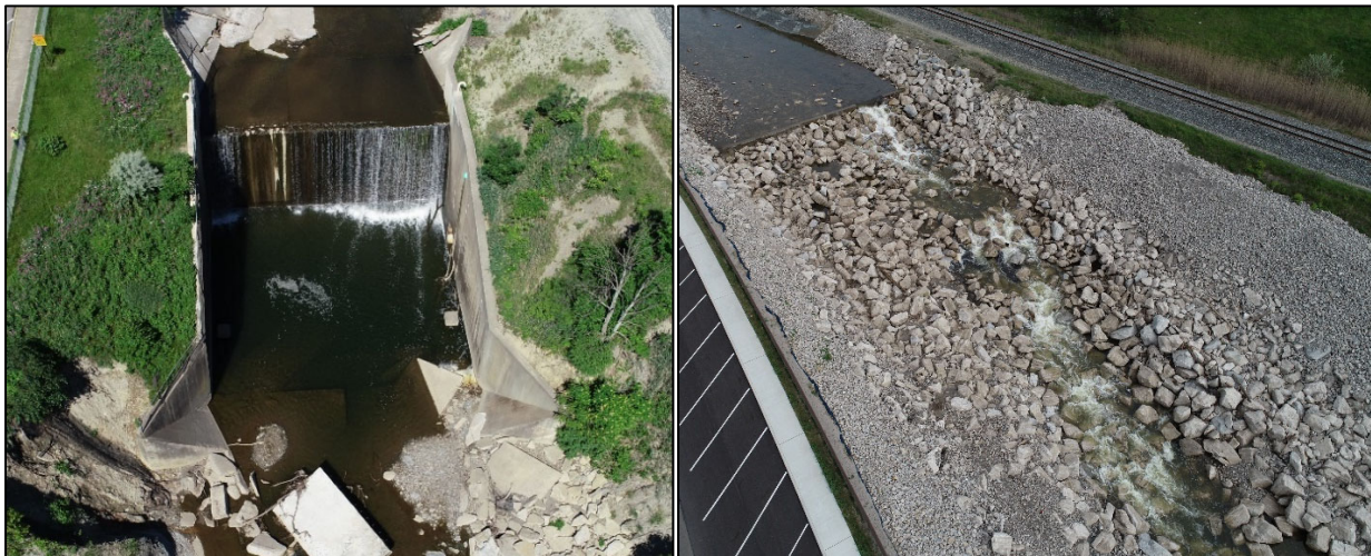
Figure 14. Big Creek 30-foot drop structure (left, 2018) and rock cascade (right, 2020) fish passage barriers.
