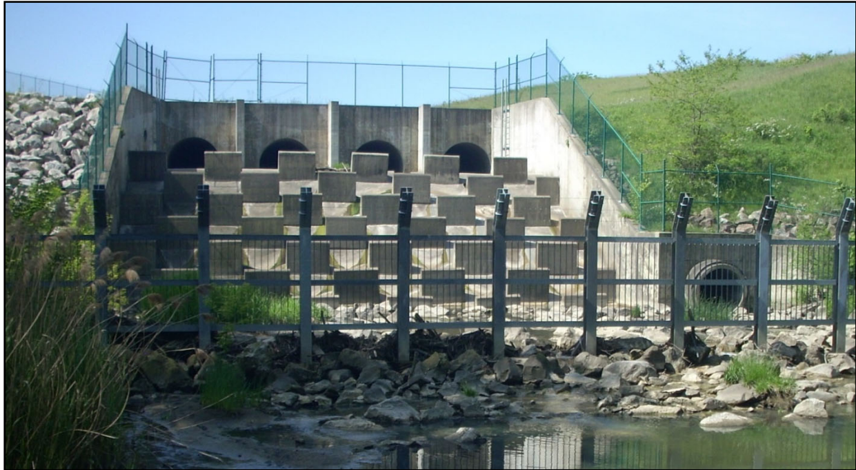
Figure 12. CHIA drop structure and culvert outlet at Abram Creek RM 1.0.
