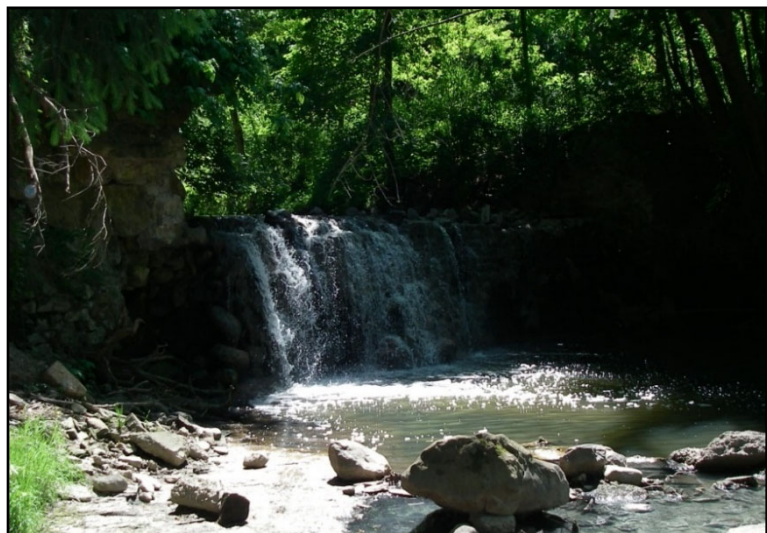
Figure 11. Low-head dam at Abram Creek RM 0.90.
