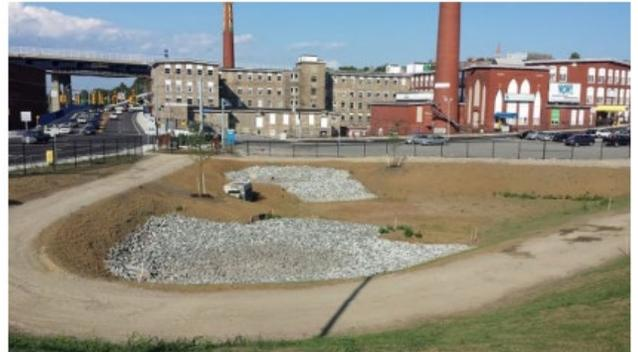
Infiltration basin in an urban area. The basin has two gravel areas for infiltration. The remainder of the basin bottom and its slopes are planted with sod. *Credit: Massachusetts Department of Transportation, taken from EPA, "NPDES: Stormwater BMP Infiltration Basin".*
