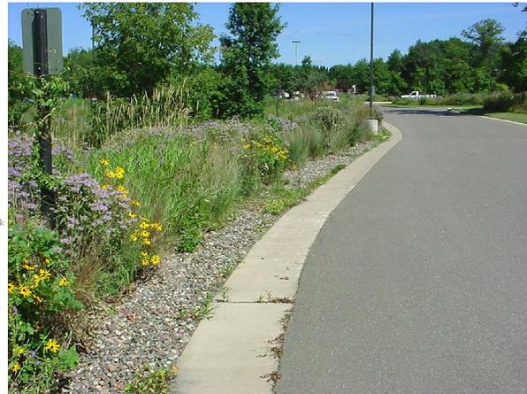
An infiltration trench in the city of Lino Lakes, MN. This design took aesthetics and environmental factors (i.e. plants for pollinators) into consideration. Credit: Minnesota Stormwater Manual, "Design Criteria for Infiltration"
