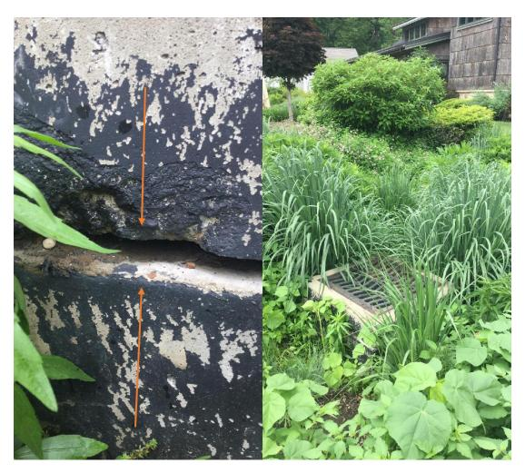
Explanation: This cracked outlet is letting flow right into the practice without proper treatment (SE corner of building).
