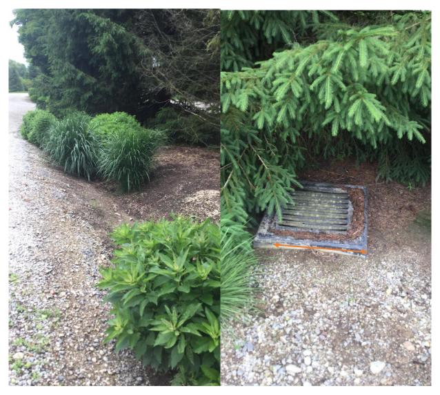
Explanation: The sediment from parking lot is flowing into this practice, potentially clogging the bioretention cell.
