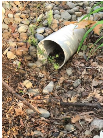
Picture 2: Debris in the Inlet Pipe of the Bioretention Pond to the North West
