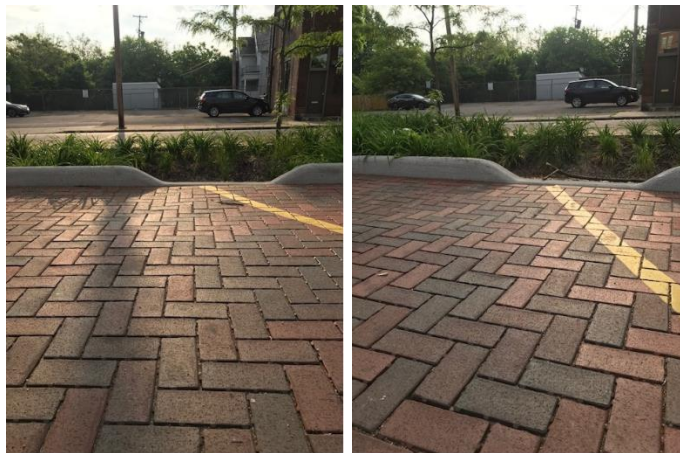
Picture 3 & 4: Low Points in Pervious Pavers to the East of the Parking Lot
