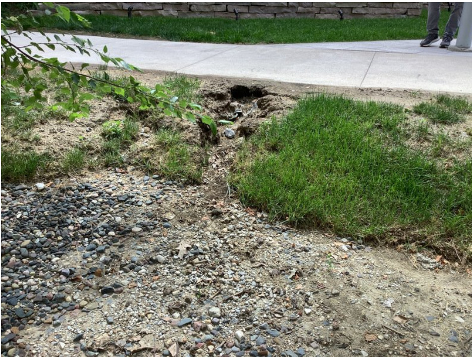
View of erosion and accumulated sediment on the north end of the bioretention cell (facing east).
