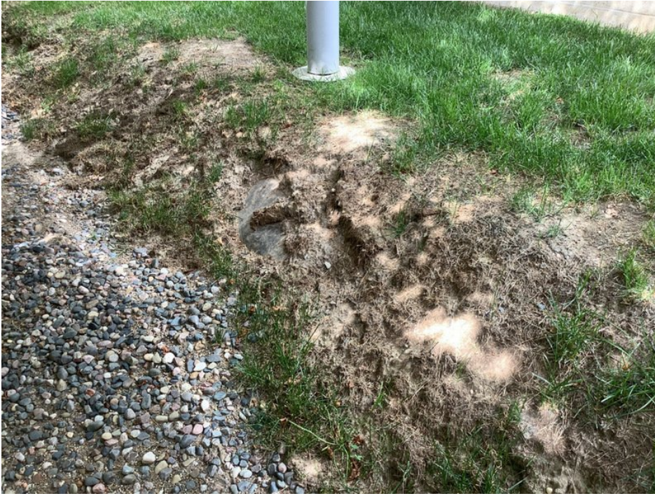
View of erosion and exposed liner on the west embankment of the bioretention cell (facing southwest).
