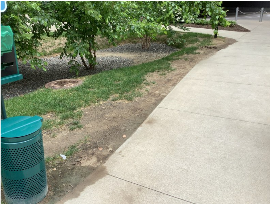
View of exposed soil along the east side of the bioretention cell (facing north).
