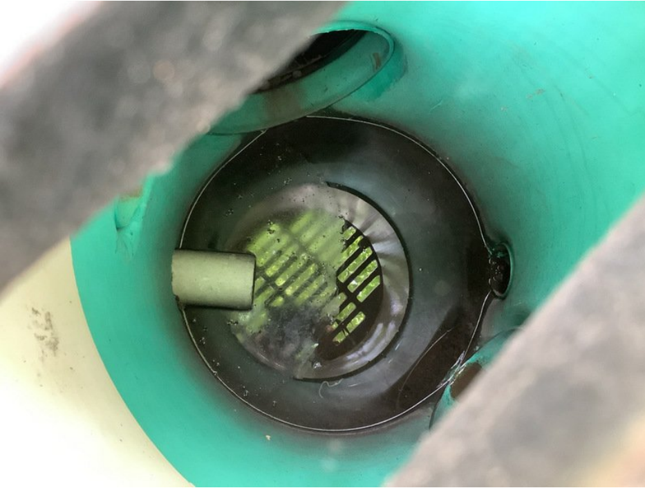
View of the interior of the bioretention cell outlet structure.
