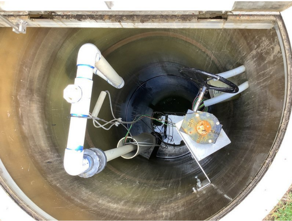
View of the interior of the manhole with water control valve for rainwater harvesting.
