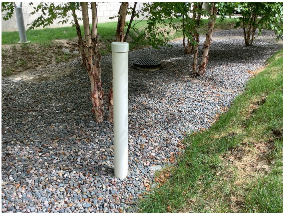
View of the cleanout pipe in the bioretention cell (facing north).
