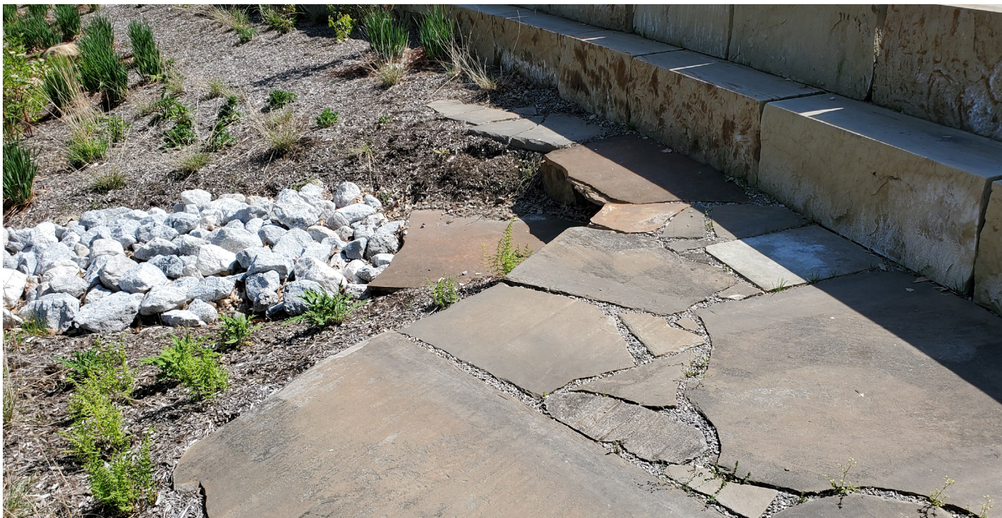
5. No erosion observed at outlet structure
