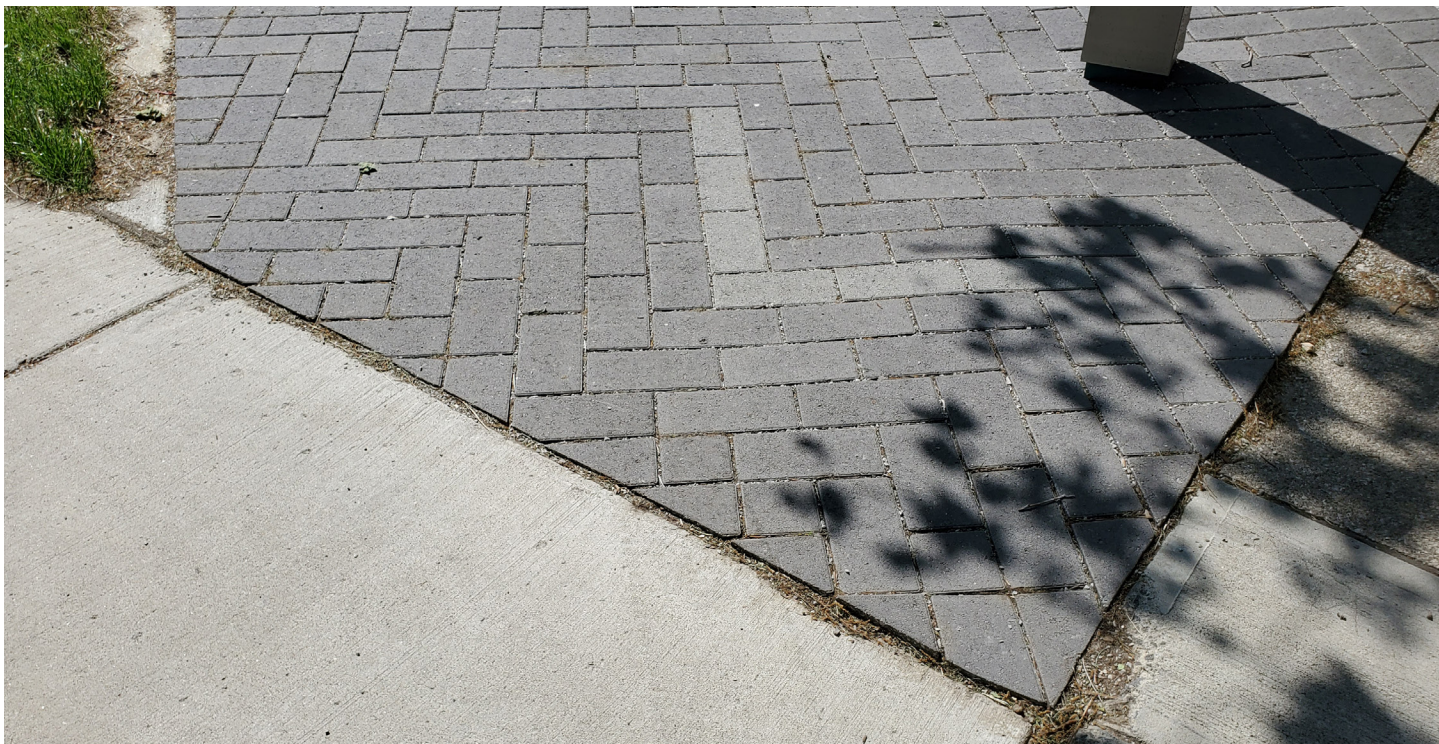
9. Minor sediment observed at corner of pedestrian walk due to unstabilized adjacent area - vacuuming scheduled
