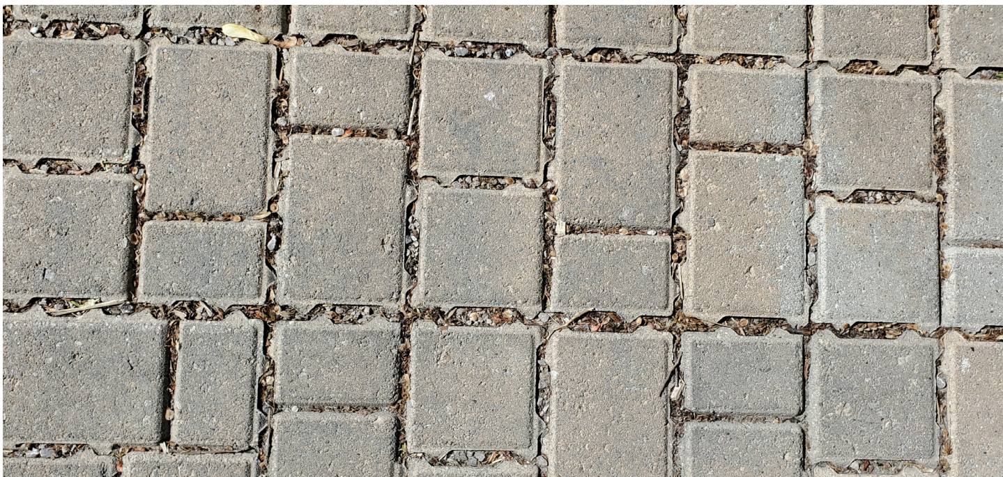
2. Permeable pavers (close-up) w/ minor debris - vacuuming scheduled
