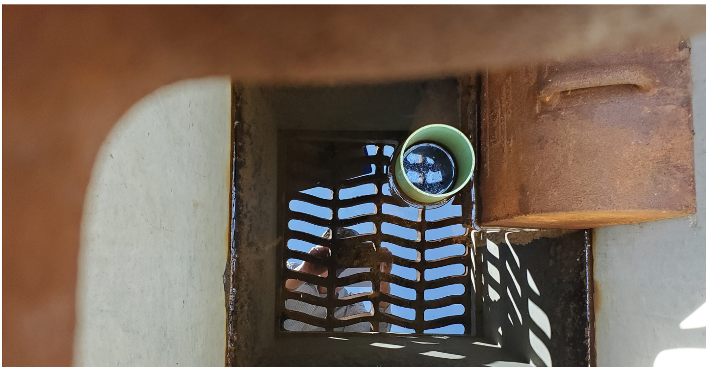
8. Bioretention outlet structure - clean, no debris
