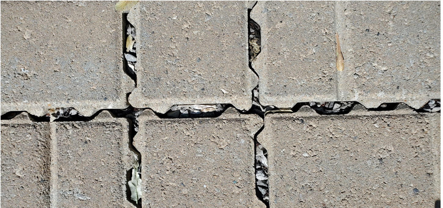
3. Permeable pavers (close-up) clean
