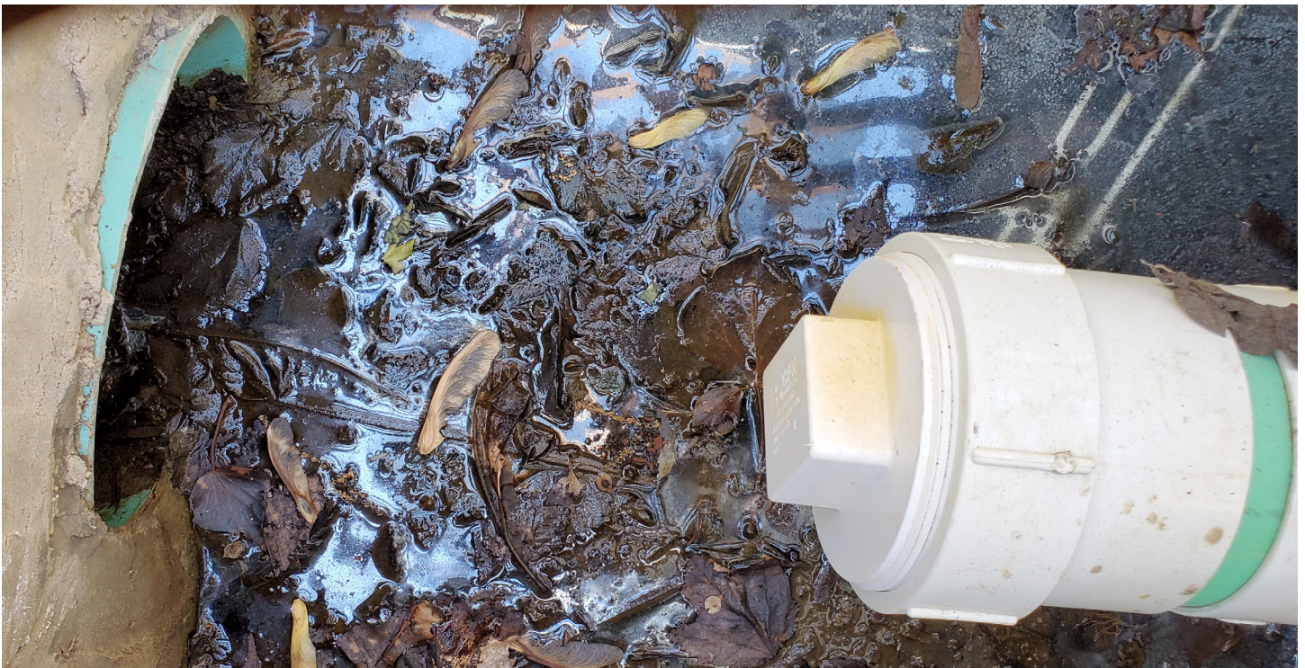
4. Permeable paver outlet structure - starting to accumulate debris (expected w/ no outlet flow) - yearly cleaning discussed with owner
