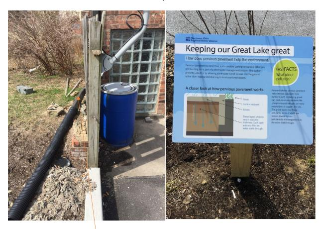
**Photo 1:** Flow is dispersed to the cell from this downspout.
