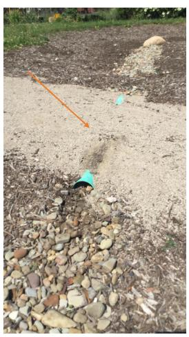
Explanation: This pipe will need to be cleaned out in order to convey stormwater correctly. (This pipe has been removed (10/31).
