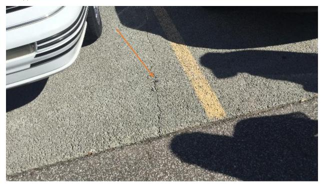
**Explanation: Minor cracking observed within the porous concrete.**
