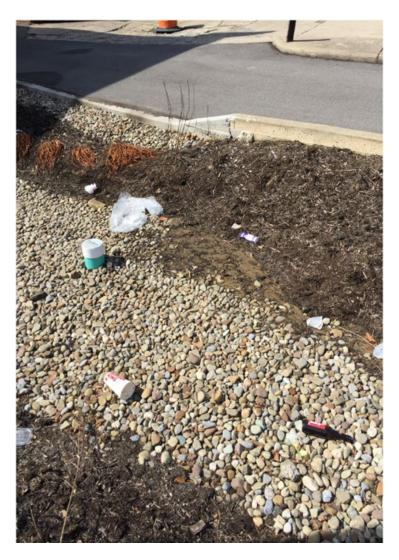
Debris has accumulated in the cell and needs to be removed. Concave shape regarding the North side of the cell behind the parking lot is recommended.
