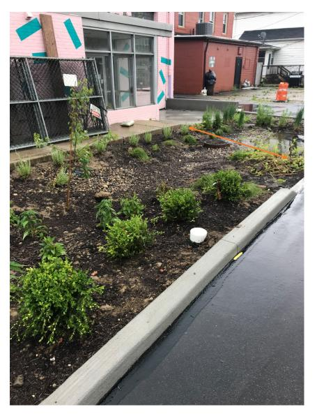
Explanation: During the inspection we noticed the matting that has been placed down has been compromised. Ensure it will not impact the function of the practice.
