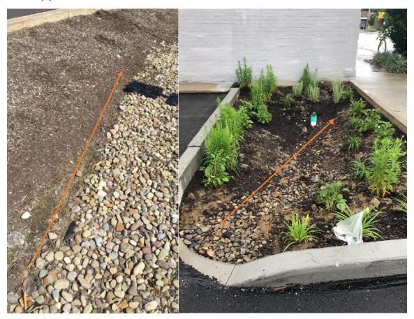
Explanation: Low flow rock channels need to be formed in a concave manner. The applicant will also need to remove debris from the practice that is at the entrance of the property. Ensure runoff is not first entering parking lot drain (just off right-hand photo) prior to entering the cell (i.e., add solid lid, re-grade as necessary, etc.).
