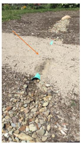
Explanation: This pipe will need to be cleaned out in order to convey stormwater correctly.
