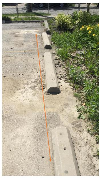
Explanation: The sediment-laden runoff from construction activity is getting into the practice and may cause further problems (e.g., clogging of soils). Applicant must ensure this will be removed and cleaned up.
