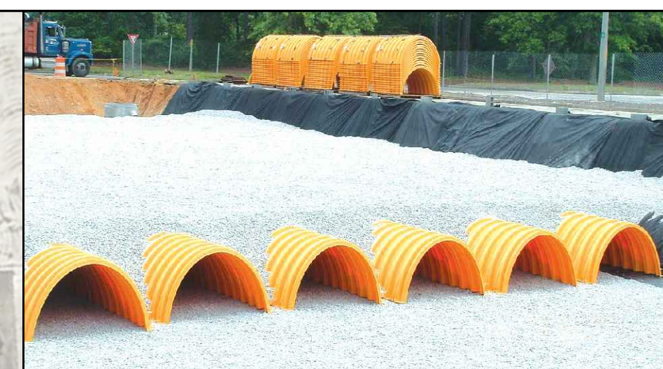
UNDERGROUND DETENTION EXAMPLE
