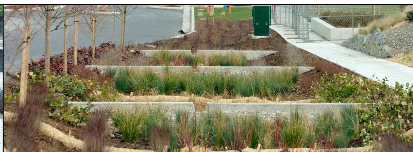
TERRACED BIORETENTION EXAMPLE
