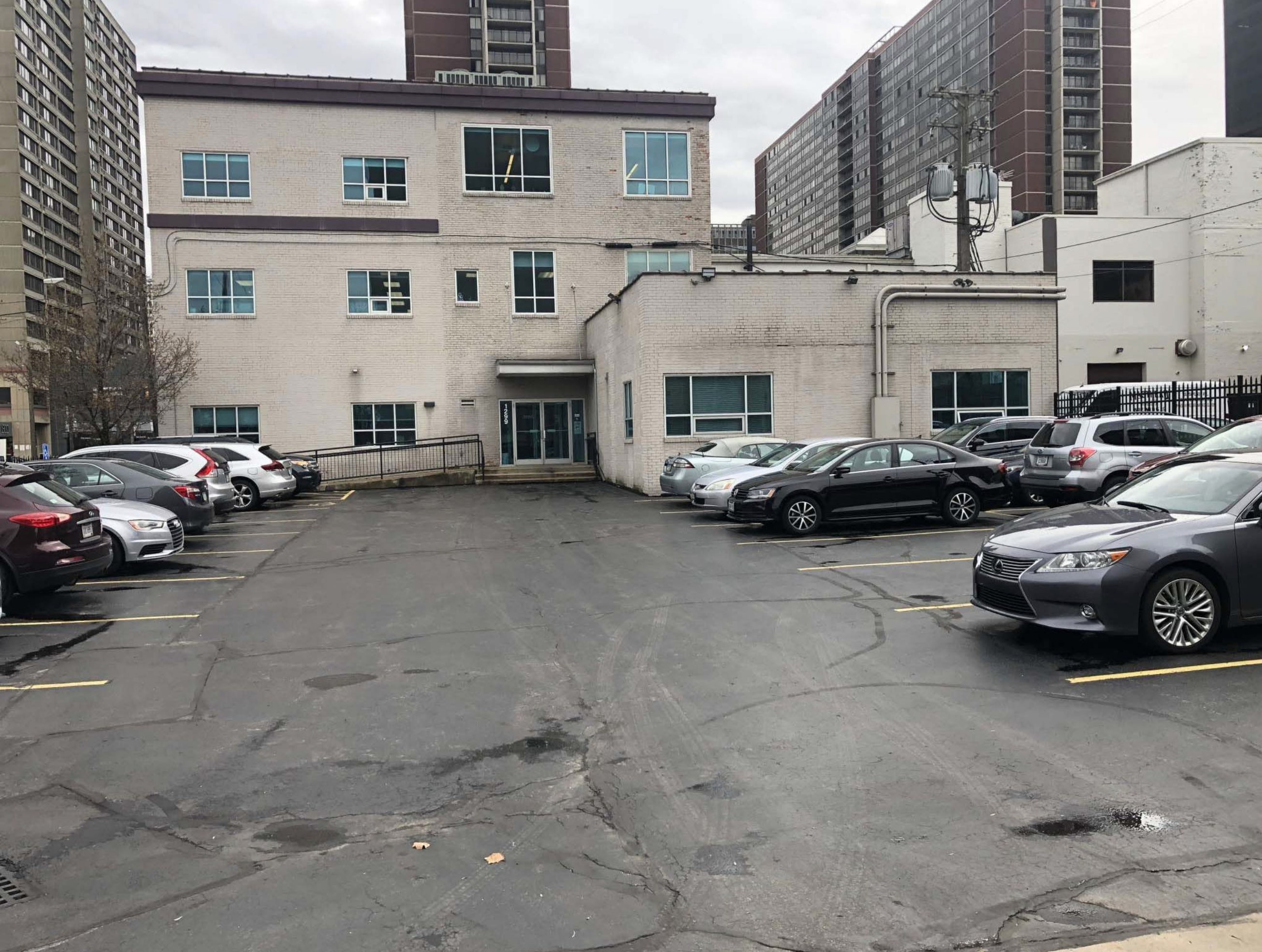
FIGURE 4 EXISTING CONDITIONS PHOTOGRAPHS
