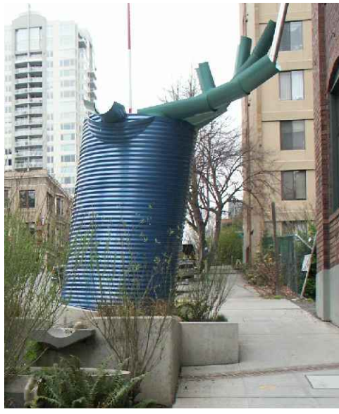
PROPOSED CISTERN (ROOF WATER)
