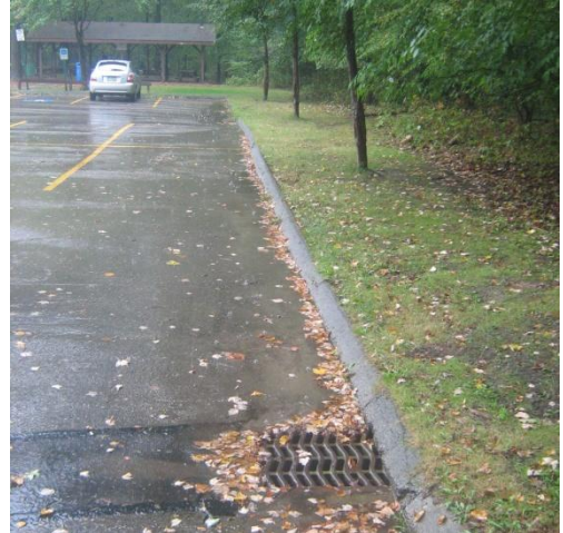
Photo #6 – East Parking Lot Looking East
