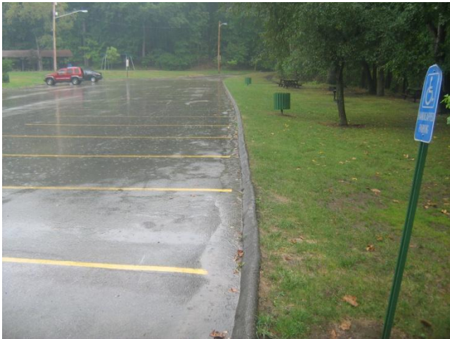
Photo #3 - West Parking Lot Looking East
