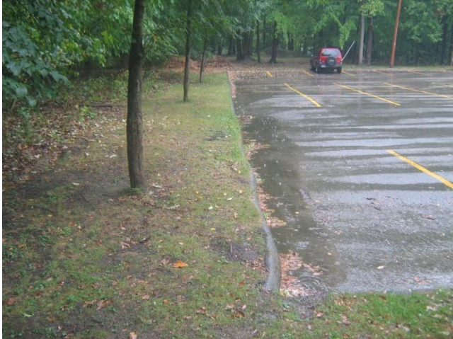
Photo #5 – East Parking Lot Looking West
