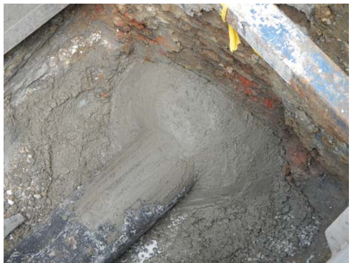
PHOTO 04: Concrete collar formed
