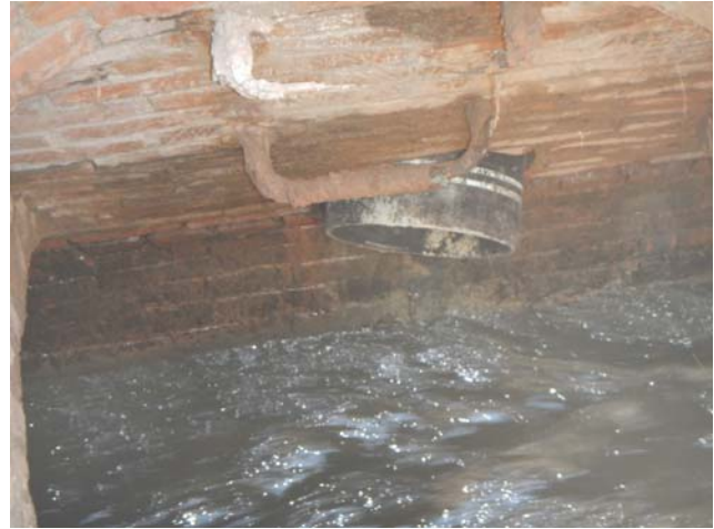
PHOTO 04: Concrete collar formed
