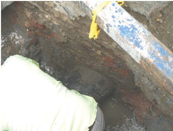
PHOTO 03: Annular space filled with hydraulic cement
