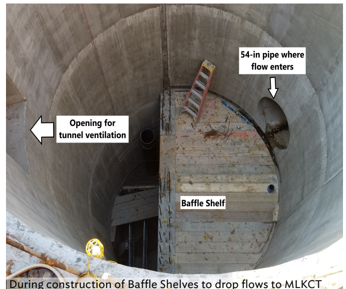
During construction of Baffle Shelves to drop flows to MLKCT
