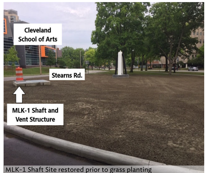
MLK-1 Shaft Site restored prior to grass planting
