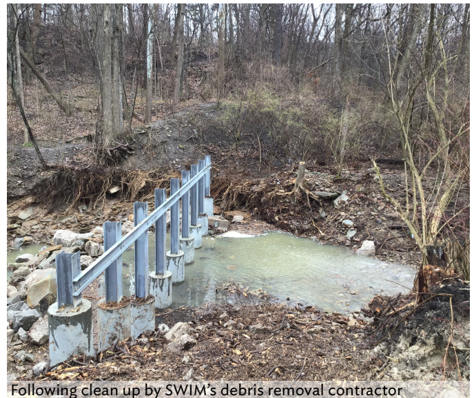
Following clean up by SWIM's debris removal contractor
