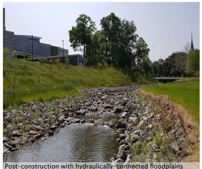
Post-construction with hydraulically-connected floodplains
