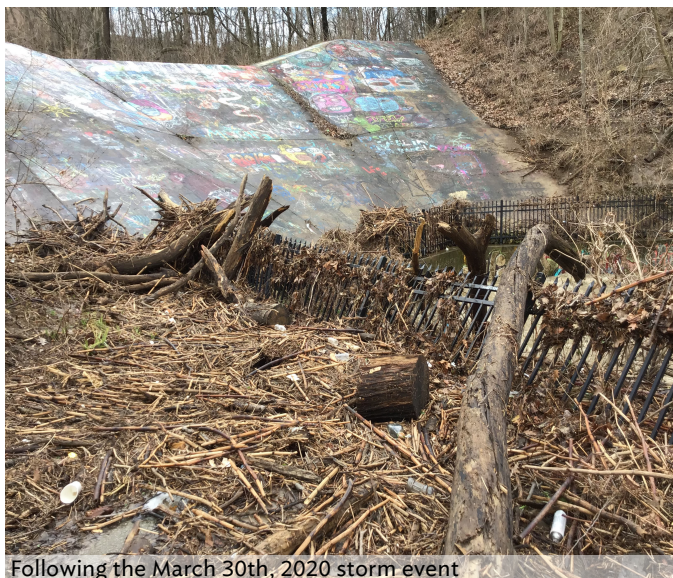
Following the March 30th, 2020 storm event
