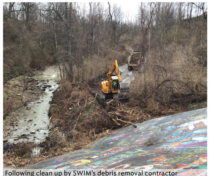
Following clean up by SWIM's debris removal contractor
