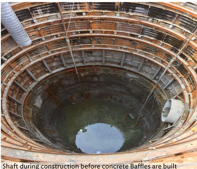
Shaft during construction before concrete Baffles are built
