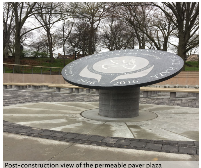
Post-construction view of the permeable paver plaza
