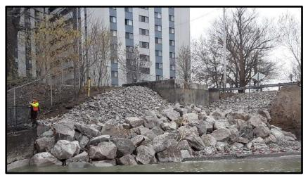
CSO-206 Emergency Repair Armor Stone Revetment Completed Spring 2020
